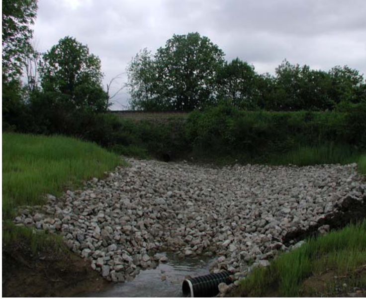
GRADE STABILIZATION STRUCTURE
