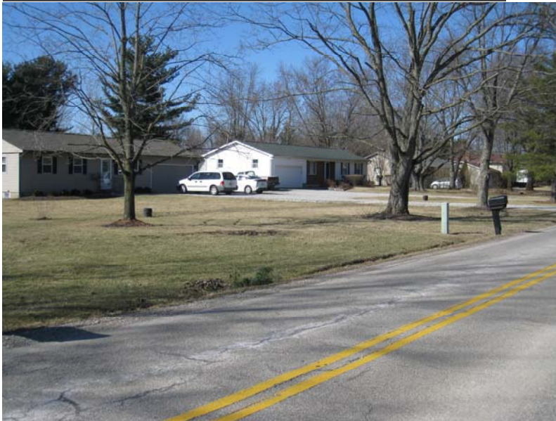
RE-SEEDING FOLLOWING SUBSURFACE DRAIN INSTALLATION
