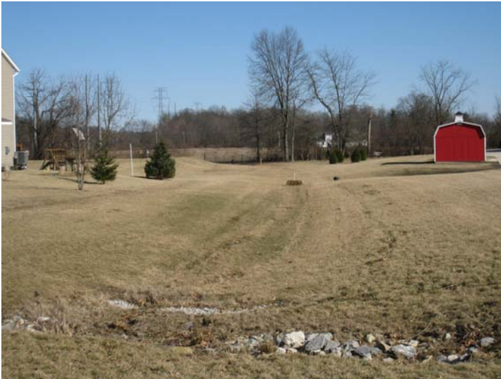
SURFACE DRAIN - SWALE
