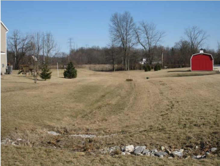
SURFACE DRAIN - SWALE
