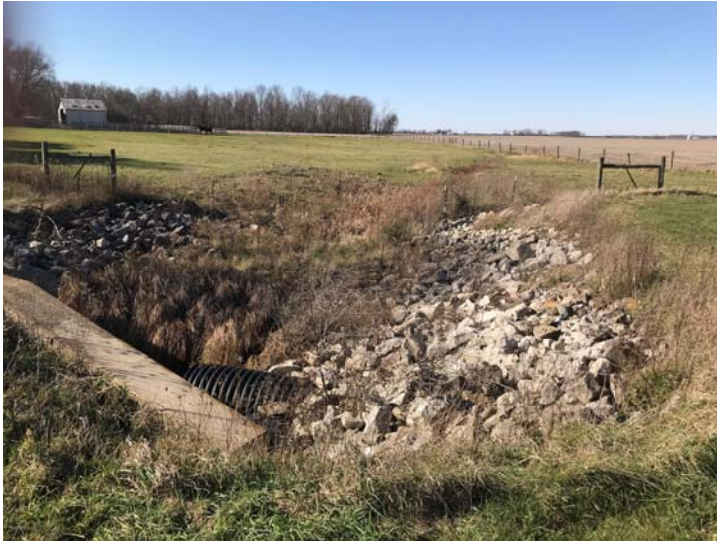
GRADE STABILIZATION STRUCTURE
